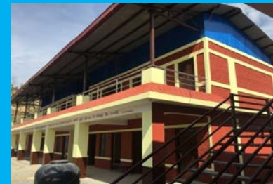
Janakalyan SS, Namobuddha- (Truss on top of RCC module)
